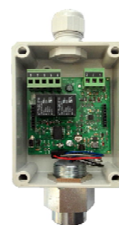
Probe with sensor remounted
