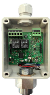
Probe with sensor to be replaced
